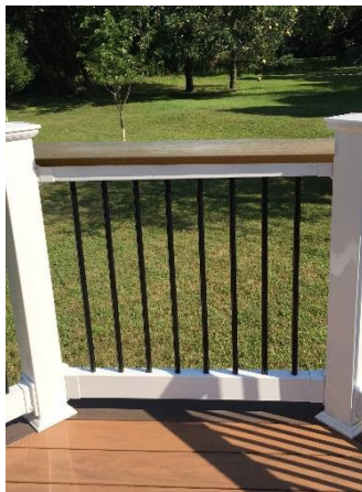
2" x 3.5" Top & Bottom Rail with ¾" Round Black Aluminum Balusters
